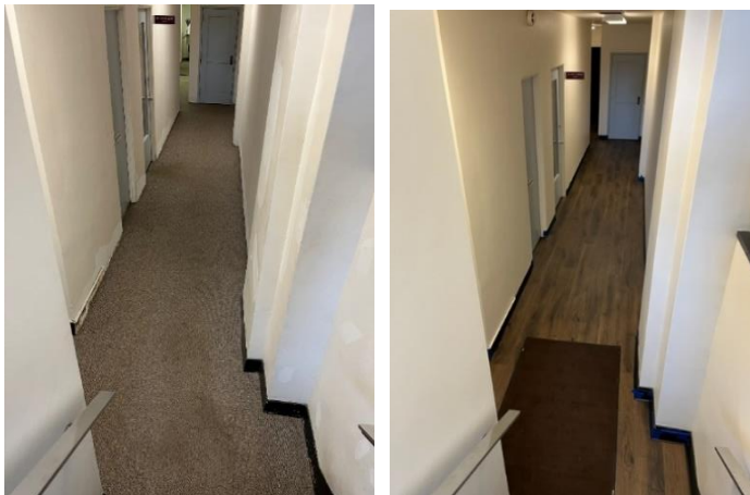
Lower level hallway
